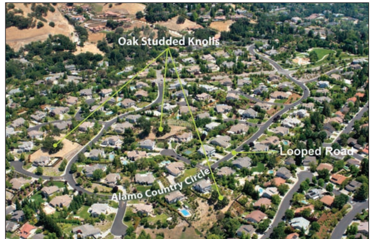
This 60 acre project, "Alamo Estates" on Alamo Country Circle, is an example of integrating a project into the natural terrain without losing density. The Alamo Improvement Association recommended approval of this project with 98 lots, because the land plan was married to the topography of the land. The project is designed below majestic oak studded knolls on the property. These knolls became significant natural features in distributing aesthetic buffers throughout the land plan.
